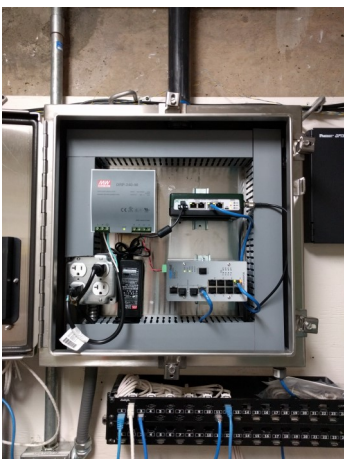
Installation at main building
