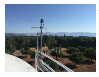
The on-site survey clearly showed that the hilly terrain of the City's Northern California rural environment prevented the reliable utilization of 900 MHz Spread Spectrum technology. A UHF 450-470 MHz system was determined to provide the most reliable results, with repeaters only required at locations where stations already existed. In the UHF band, every single station reached a signal strength of -80dBm or better.
